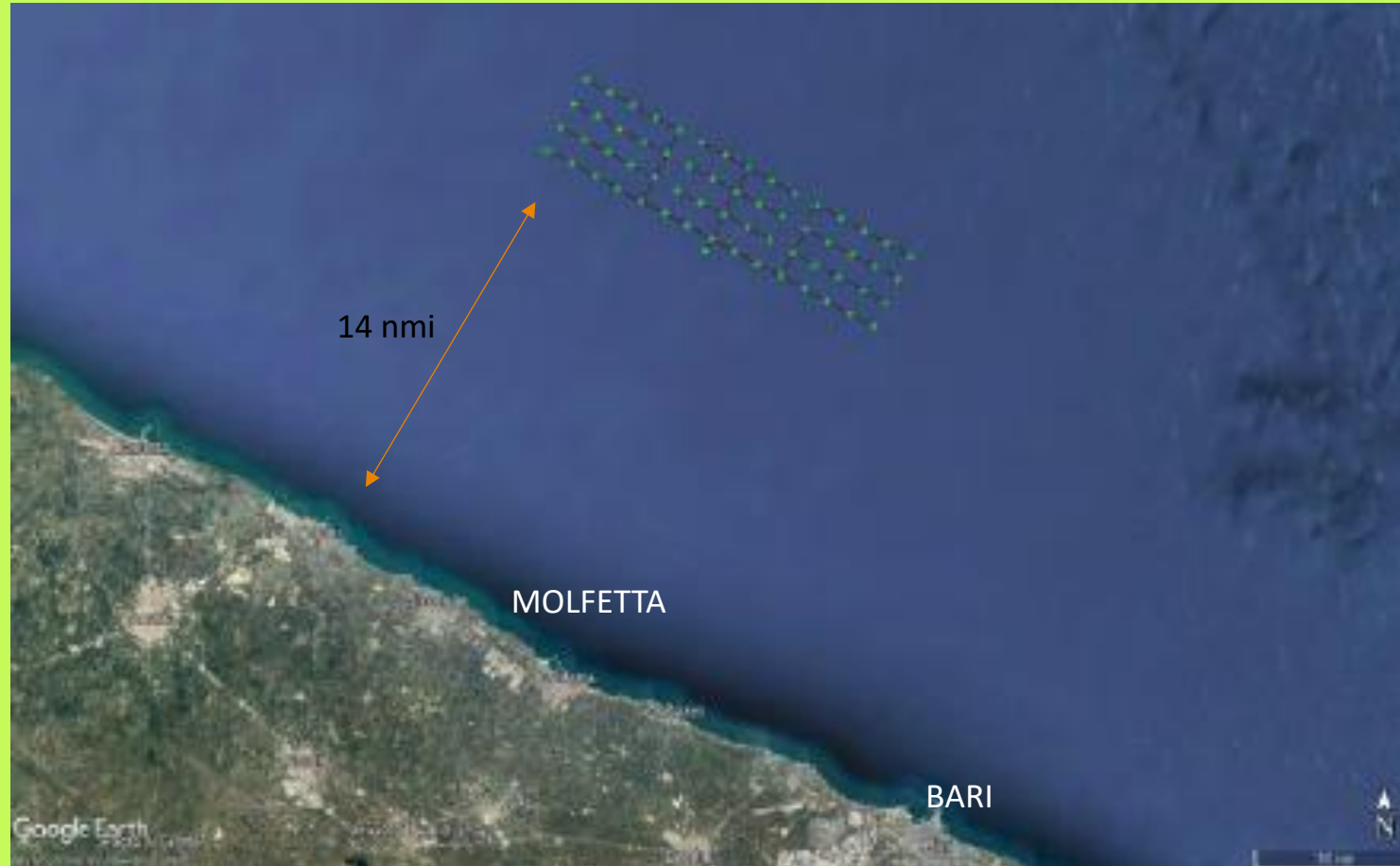
Aerial overview of the floating wind farm
